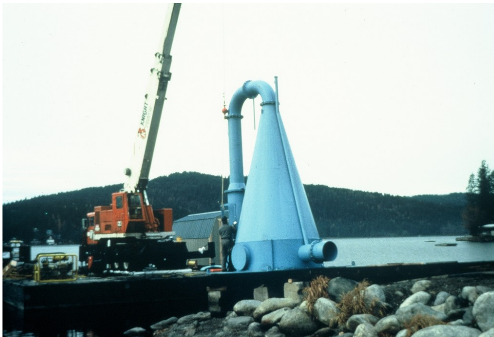
Figure 4-1 Speece Cone Being Installed in Newman Lake (from www.eco2tech.com )
